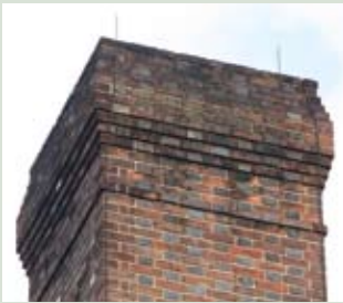
Above: A close-up of down conductor installed for this church shows how inconspicuous lightning protection can be when properly installed.
