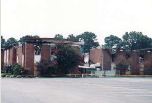
Above: Lightning fires commonly start in the steeple, roof or attic. A direct lightning strike destroyed the entire roof of this church in Mechanicsville, Virginia.
